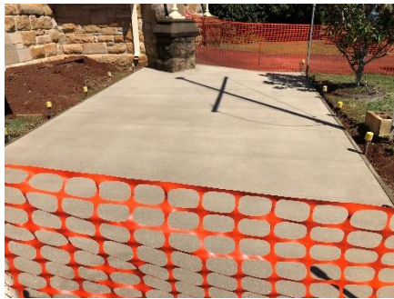
Slab outside front door of church
